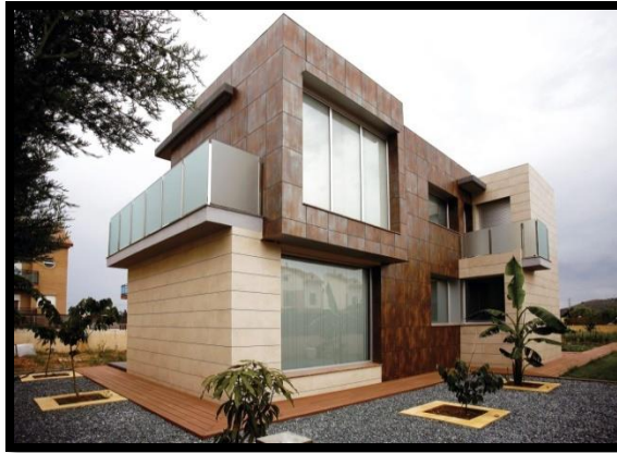
Figure No. (2) Facade of a building made of ceramic tiles with an engineering technique
