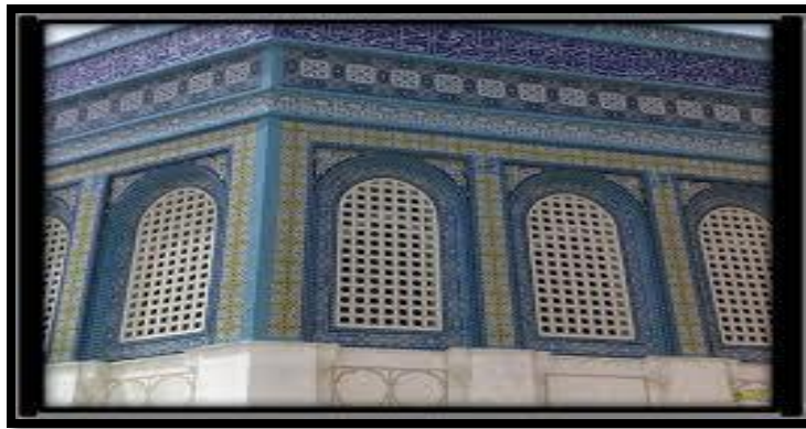
Figure No. (1) Employing ceramic tiles to show the colors of the facades of buildings/ Kairouan Mosque - Iran
